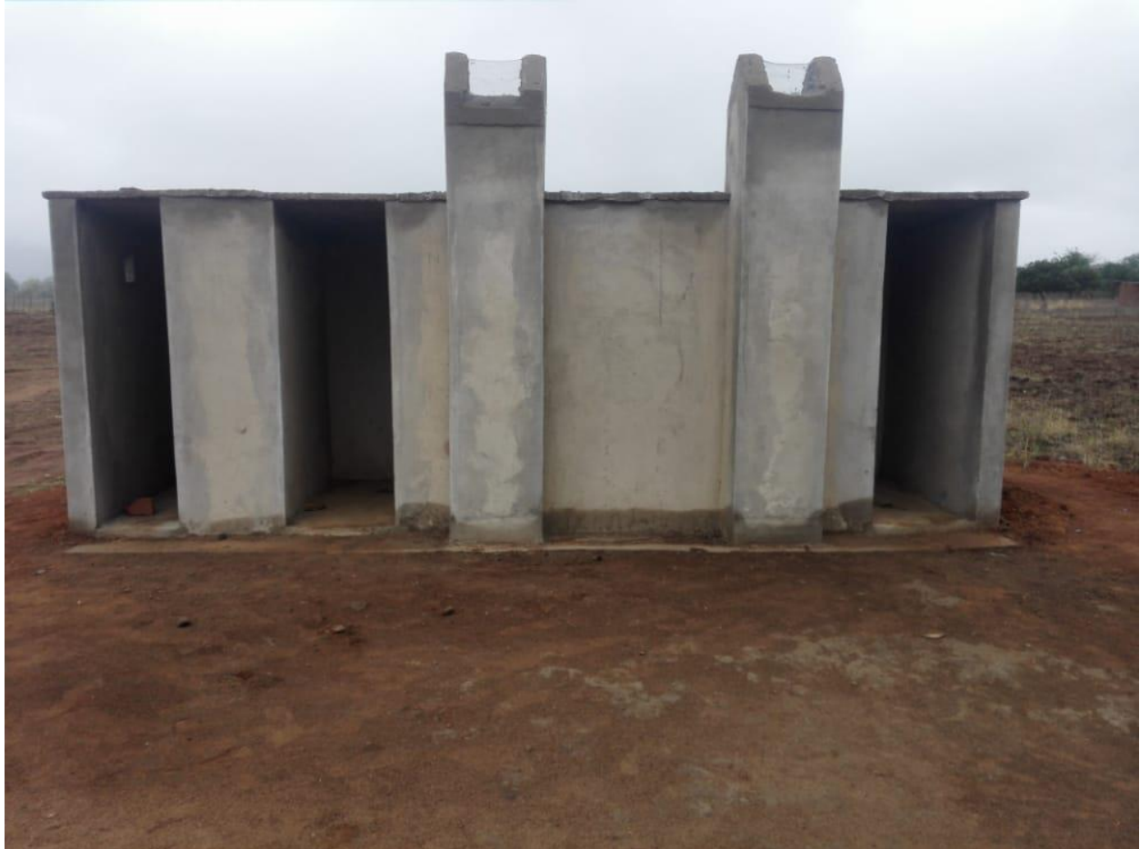
One of the BVIP latrines being constructed at Banga Irrigation Scheme
