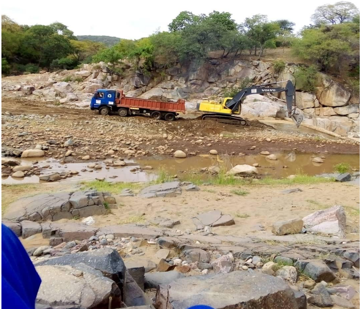
Weir Desilting- Nyanyadzi Irrigation Scheme -Manicaland Province
